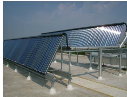
Solar Collector – Hot Water
