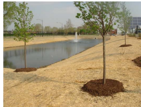
Onsite Storm Water Detention Pond
