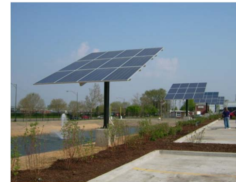
PV Electric Panels
