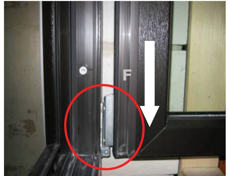
Tensile and shear forces at the corner pivot
